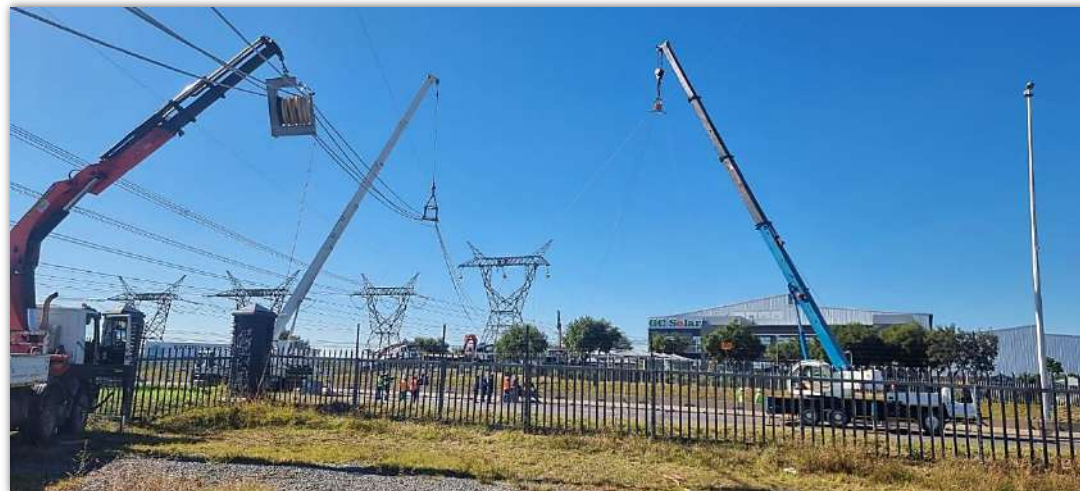
Stringing & Regulating over the N1 National Highway
